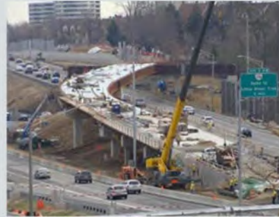
I-95 HOV/ HOT Lanes Project, Virginia
