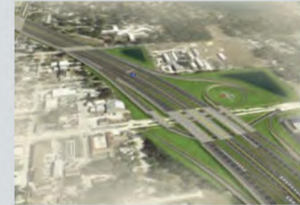
I-4 Ultimate Project, Florida
