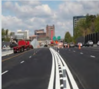
I-495 Capital Beltway HOT Lanes, Virginia
