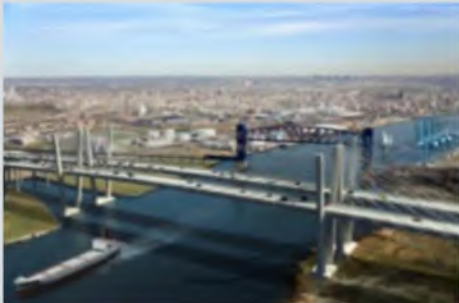
Goethals Bridge Replacement, New York, New Jersey
